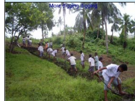
School children digging a new water supply line
