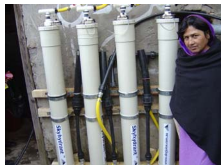
SkyHydrant Installation in Bagh
