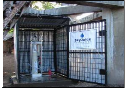
The SkyHydrant is secured in a steel enclosure to ensure that this valuable equipment is safe and ready for use
