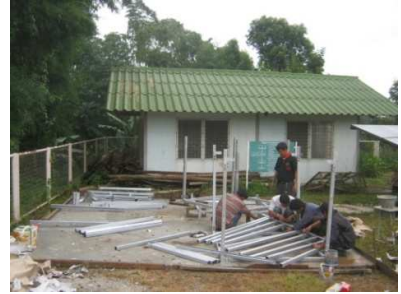
The community had laid the foundation before we arrived!
