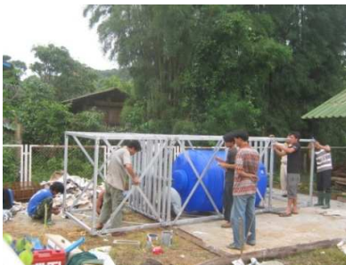
Working together to lift it upwards
