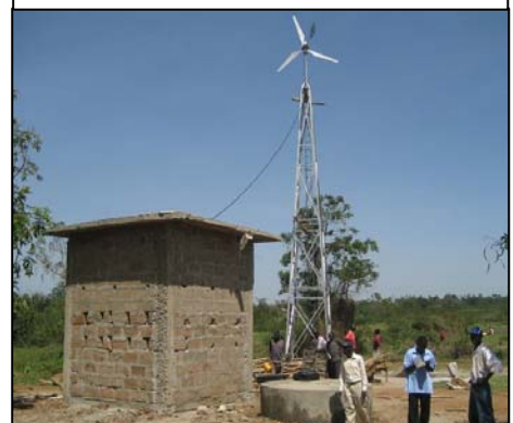
Wind generator powers the pump to draw water from Gona dam
