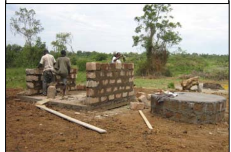
Construction of Safe Water Kiosk
