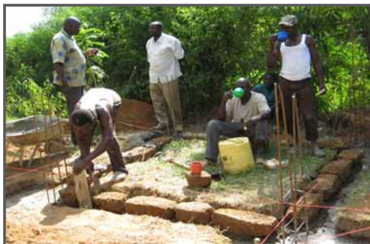
Starting the construction of the kiosk
