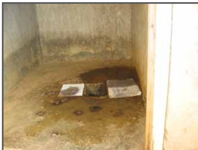
Ochilo's Primary School latrine
