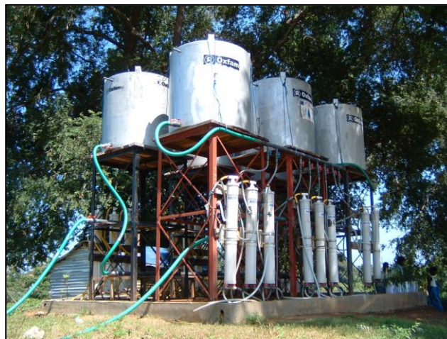
Multi Bank SkyHydrants™ Photo courtesy Oxfam GB
