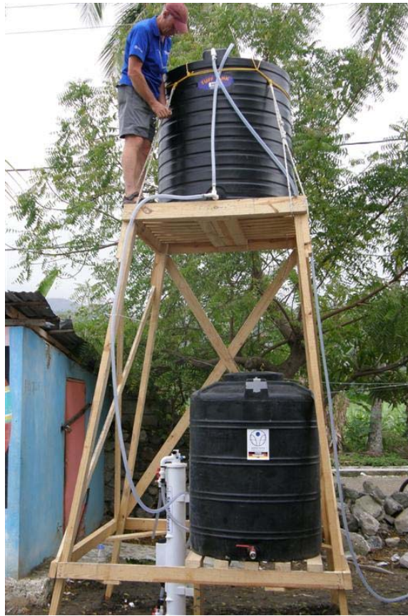
SkyHydrant with water tower
