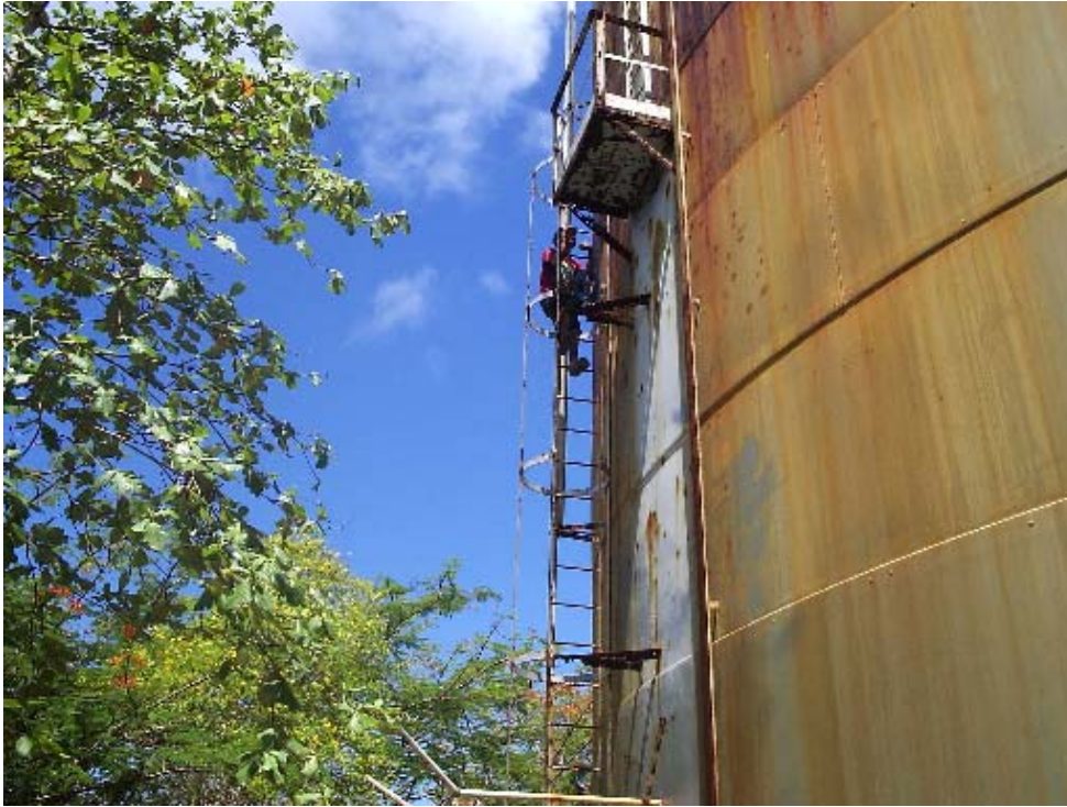
Fig. 2. Large 4,500 m 3 water storage tank (one of three) used during the phosphate exporting period from Banaba. These tanks were filled from water shipped in by the phosphate boats. There is still water in these tanks but it is red from iron oxides and people do not use it.
