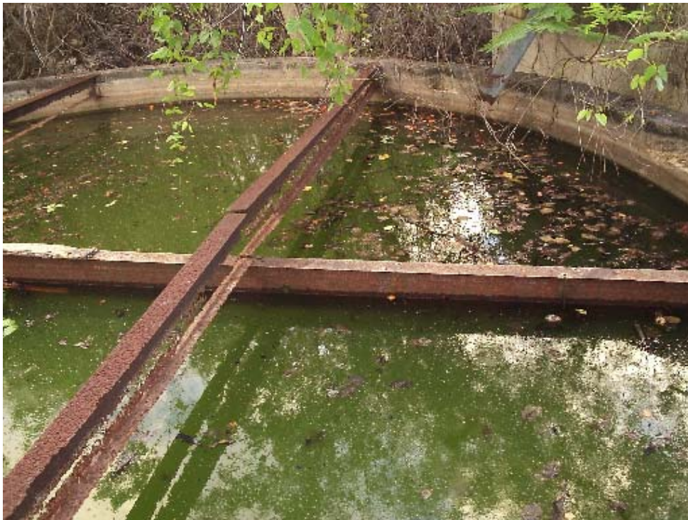
Fig. 3 Ferrocement rainwater collection tank in Banaba with algal blooms resulting in unuse of the water (Photo Moiua, WEU, MPWU).
