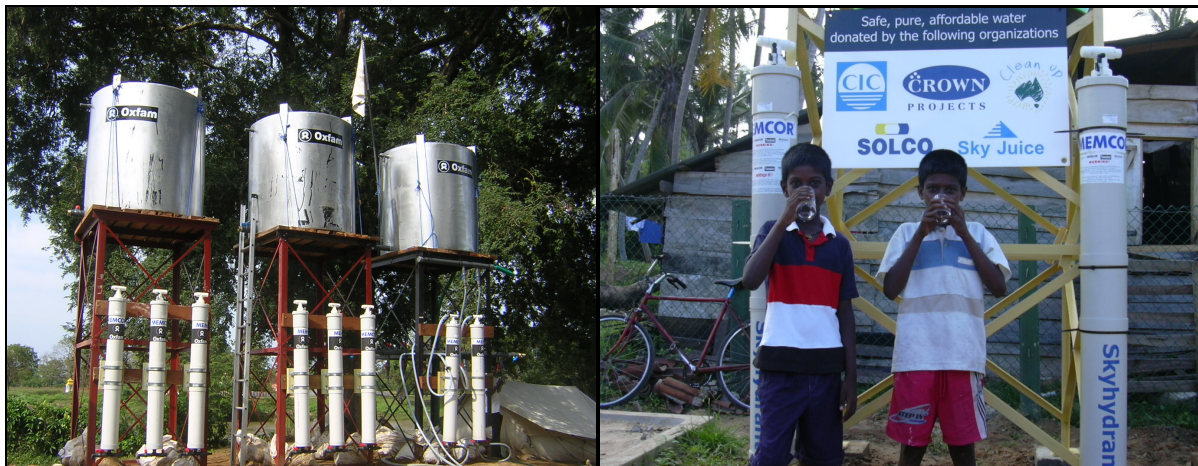
Figure 1 :Installations undertaken in Sri Lanka : Left OXFAM IDP camp installation at Batticola (100,000 L/d capacity) and a Crown Projects Skystation solar site in Seenigama (20,000 L/d capacity)
