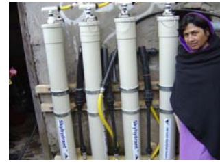
SkyHydrant Installation Bagh
